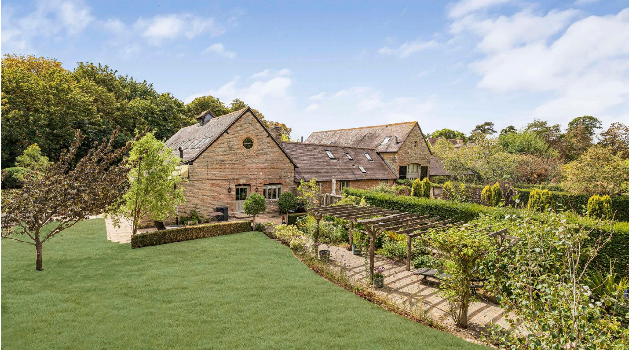
Barrow Elm Barns, Netherton, Quenington, Cirencester, Gloucestershire, GL7 5DE
